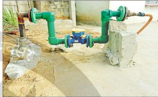
Deployment of Dhaara Smart Flowmeter at Industrial setup
